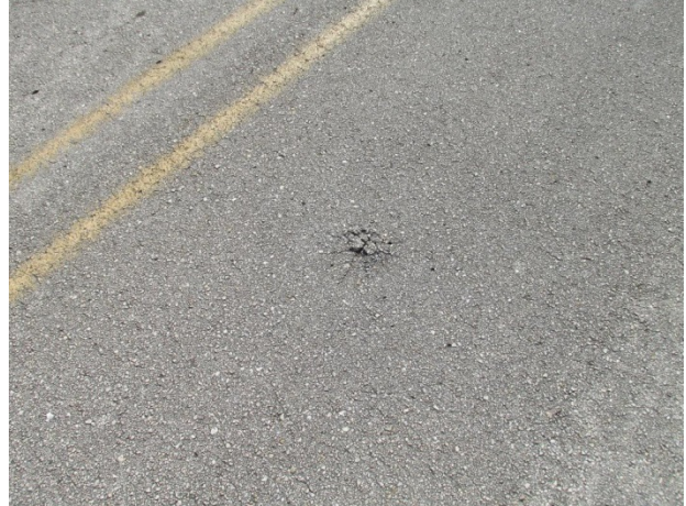
Asphalt pavement with damage evident
