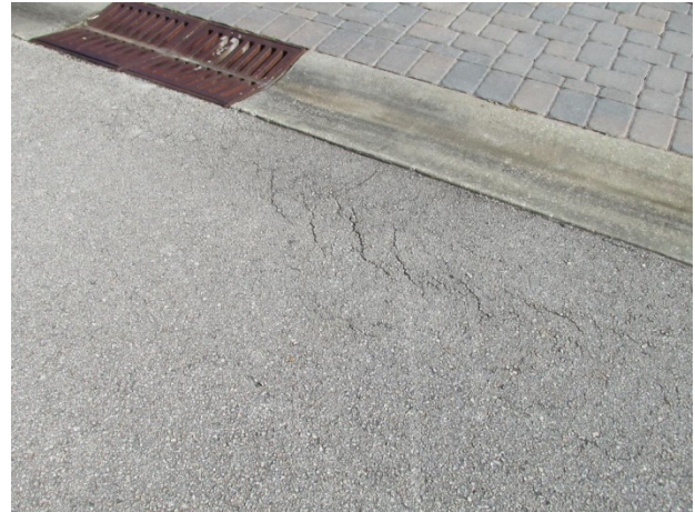
Slippage cracks evident adjacent to catch basin
