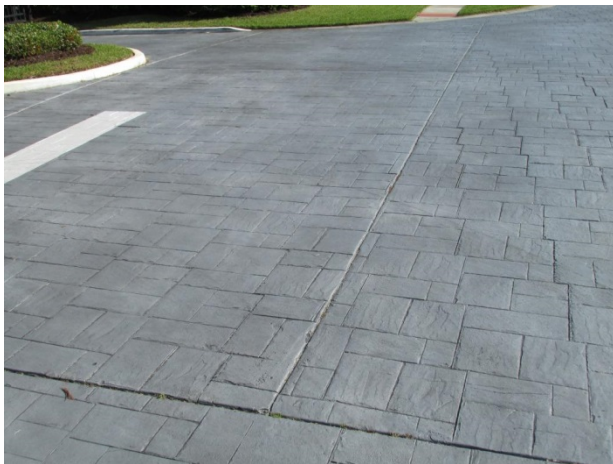
Stamped concrete streets
