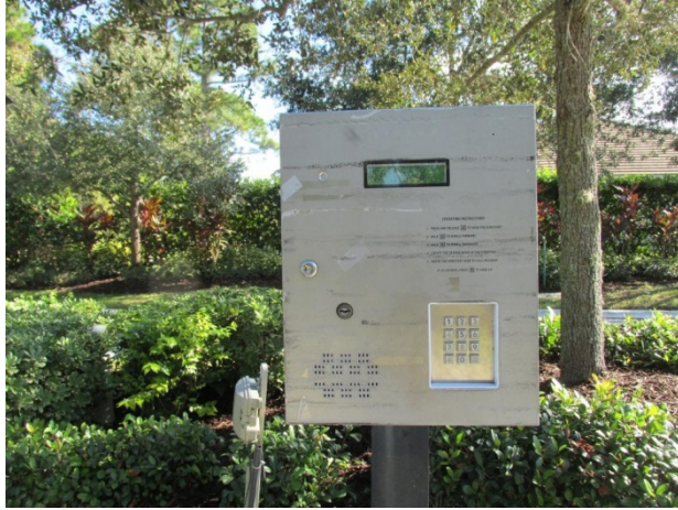
Gate entry system panel
