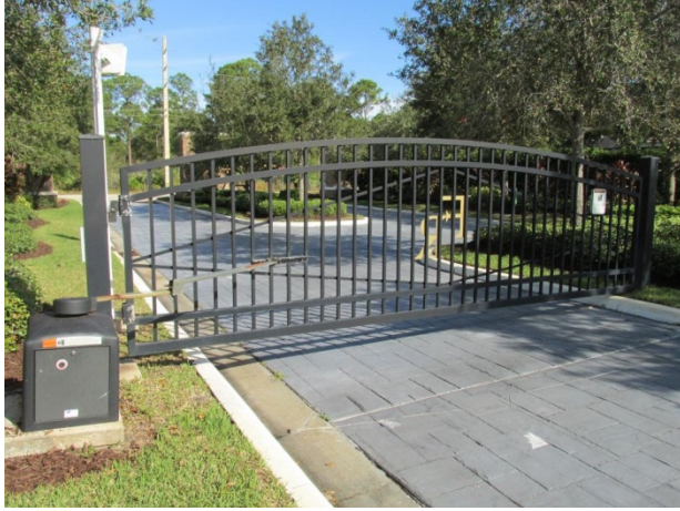
Gate and operator at front entrance
