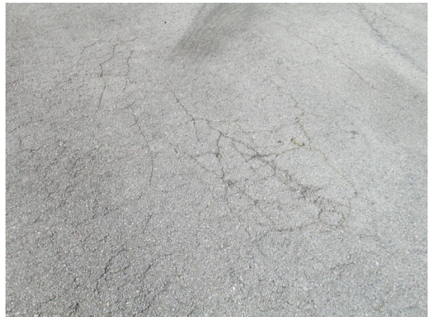
Asphalt pavement with alligator cracks evident
