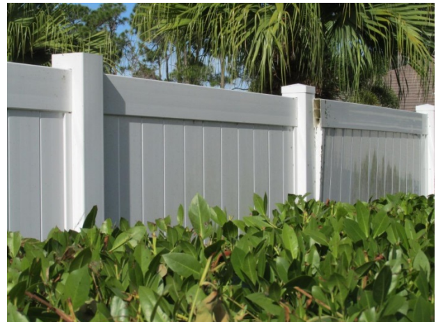
Vinyl fence with loose panel evident
