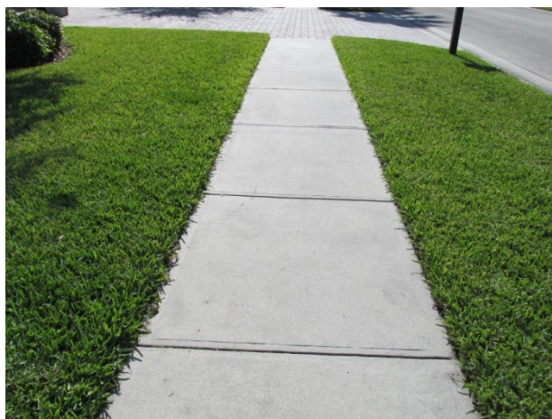
Typical concrete sidewalk
