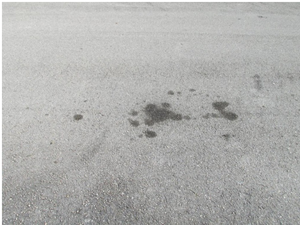
Asphalt pavement with stains evident
