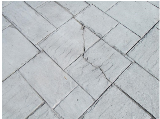
Stamped concrete streets with cracks evident
