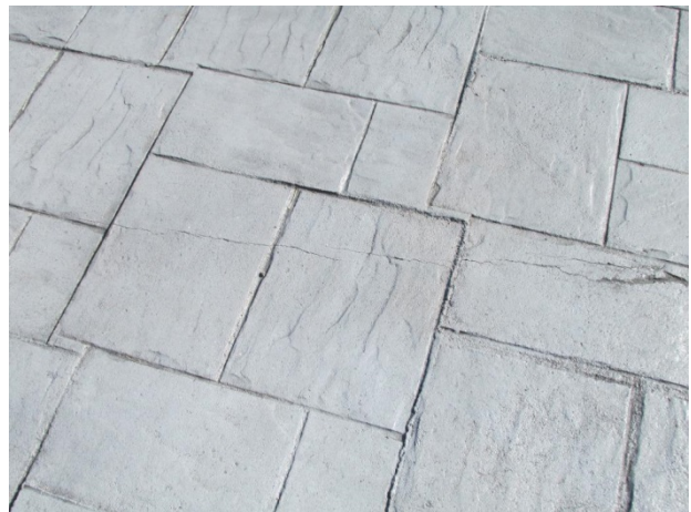
Stamped concrete streets with cracks evident
