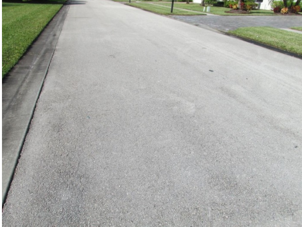
Asphalt pavement overview
