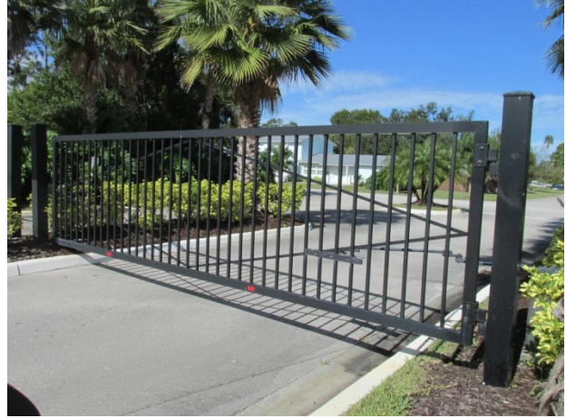
Gate and operator at rear entrance
