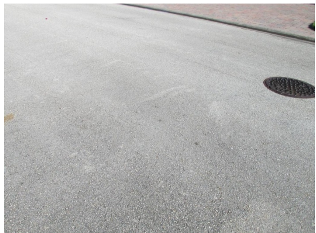
Asphalt pavement with uneven areas evident
