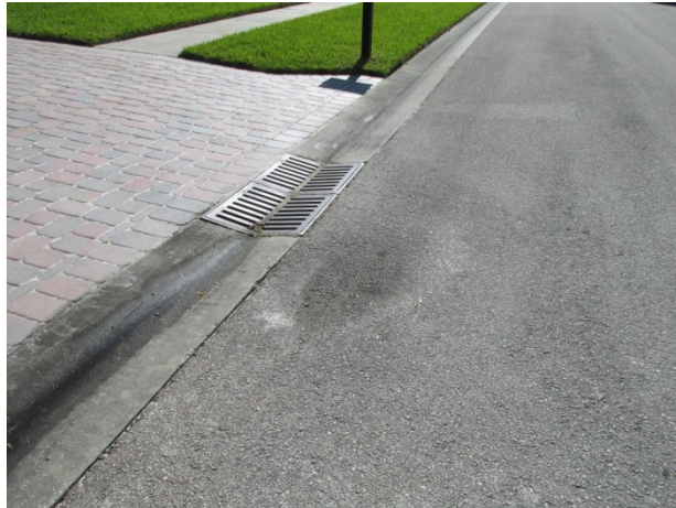
Settlement evident at catch basin
