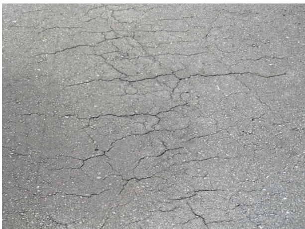
Asphalt pavement with alligator cracks evident
