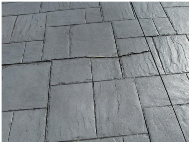
Stamped concrete streets with cracks evident
