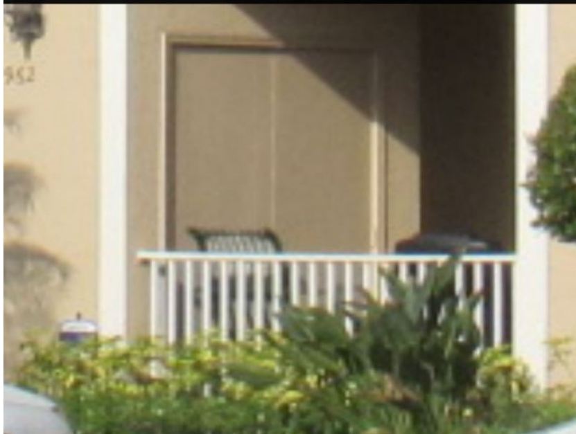
Unprotected Solid Entry Door
