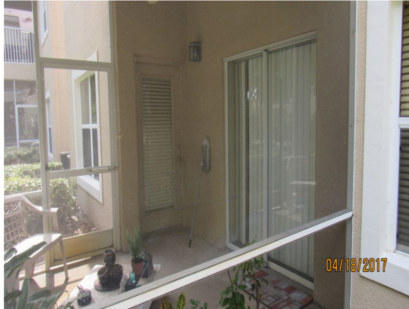
Unprotected Glazed Entry Door
