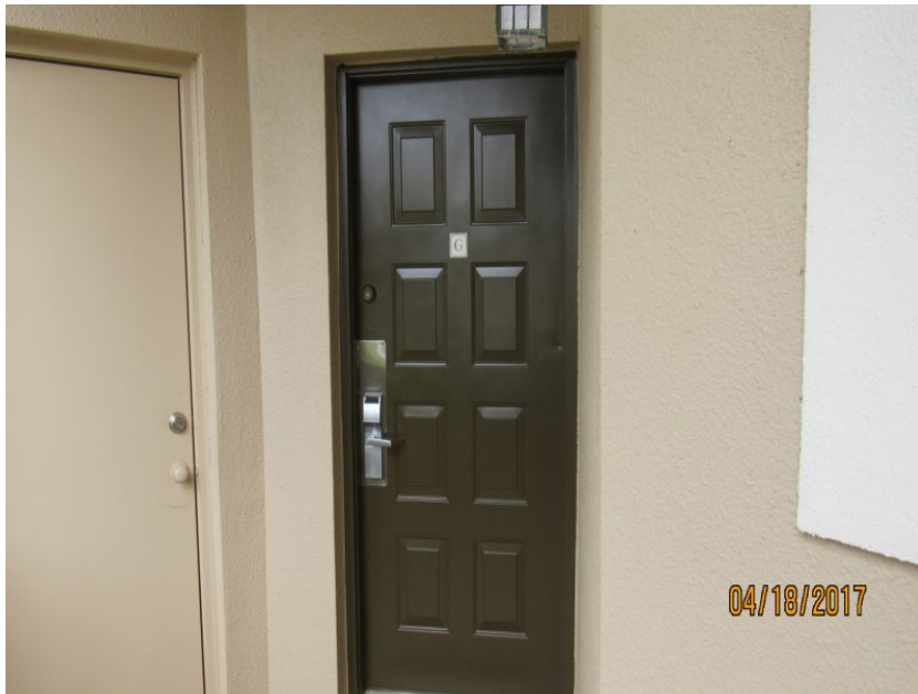
Unprotected Solid Entry Door
