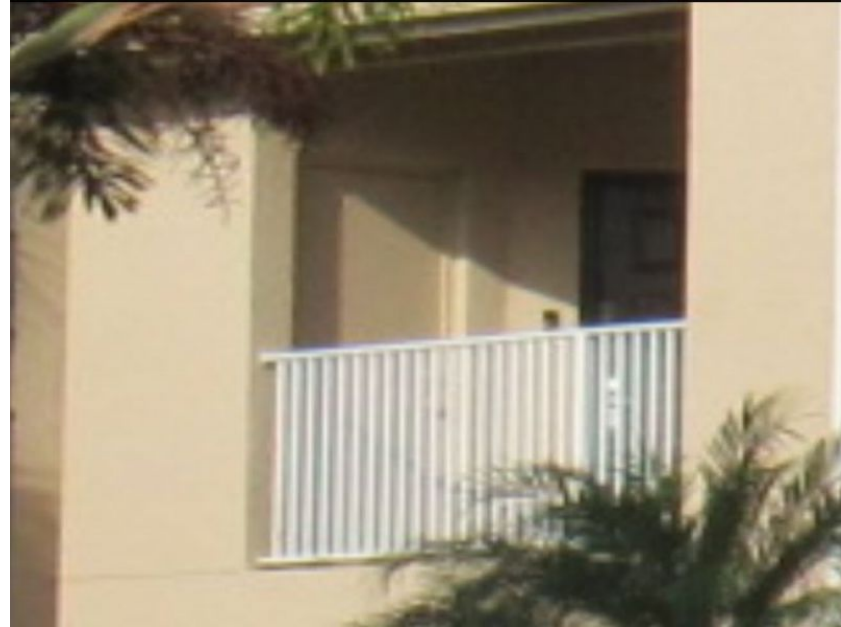
Unprotected Solid Entry Door
