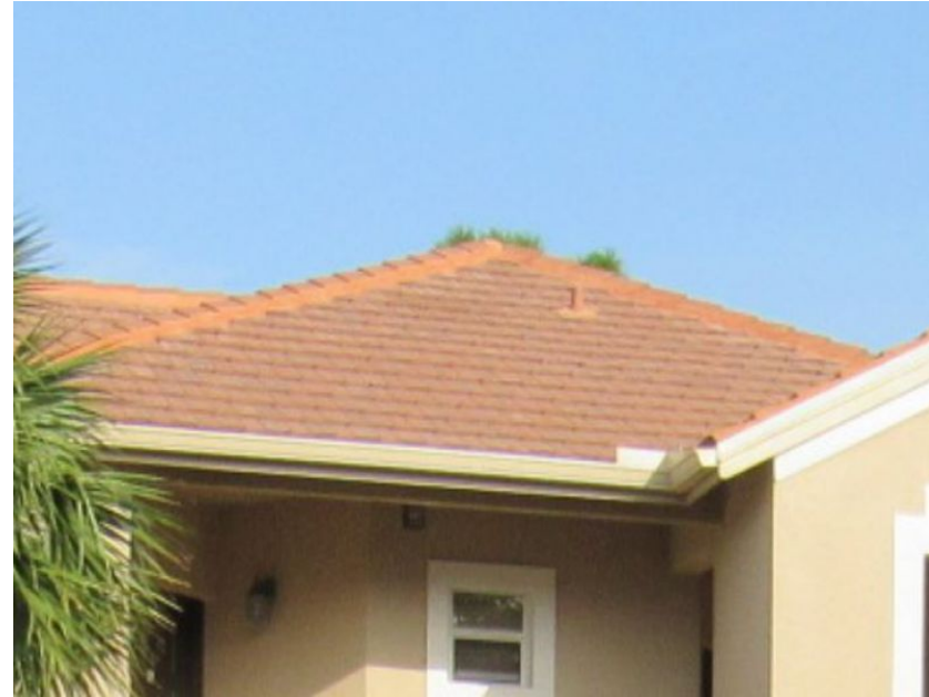
Concrete/Clay Tile Roof Covering
