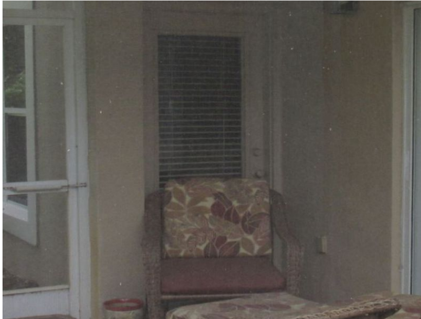
Unprotected Glazed Entry Door
