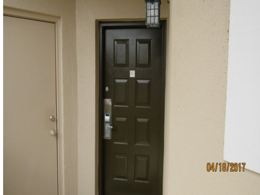
Unprotected Solid Entry Door
