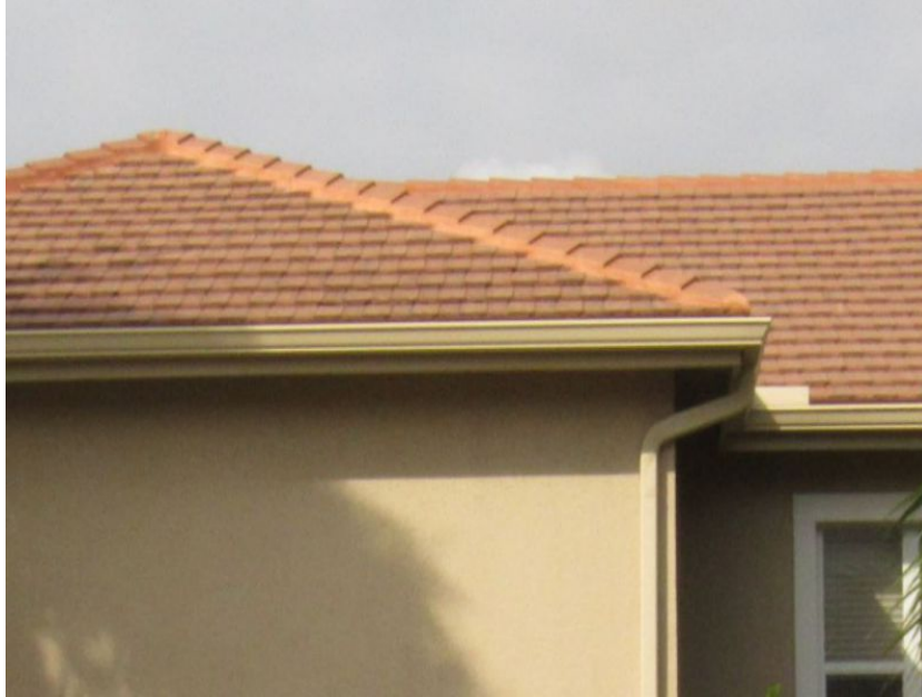
Concrete/Clay Tile Roof Covering
