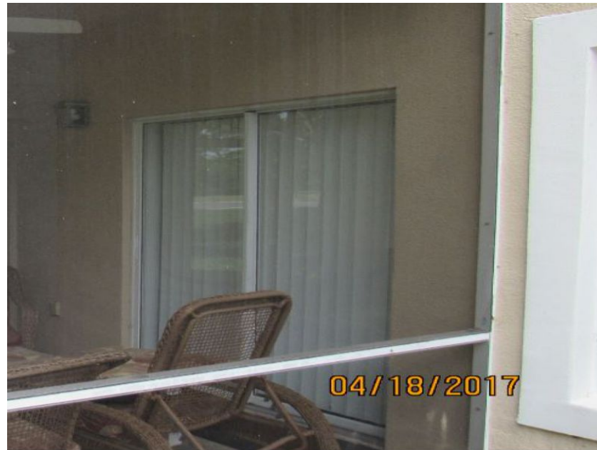
Unprotected Glazed Entry Door
