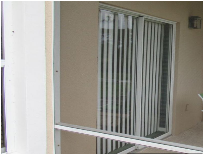
Unprotected Glazed Entry Door
