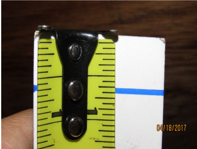
5/8" Deck Thickness Confirmed
