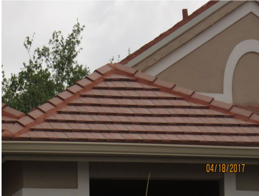
Concrete/Clay Tile Roof Covering
