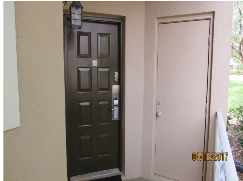
Unprotected Solid Entry Door
