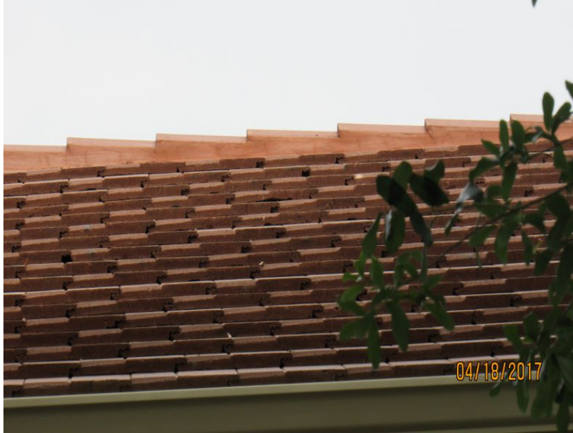
Concrete/Clay Tile Roof Covering
