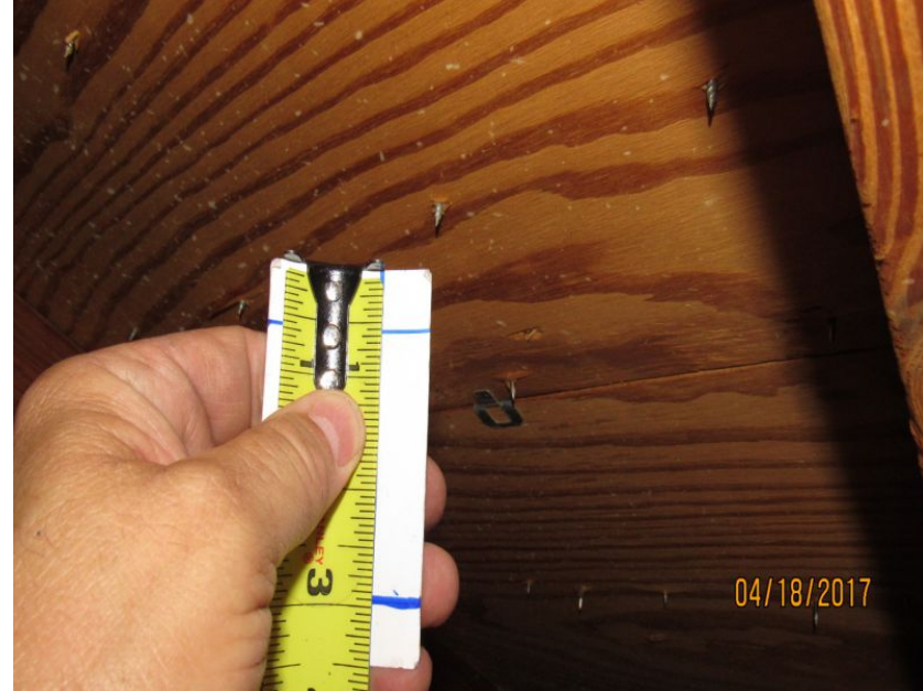
5/8" Deck Thickness Confirmed
