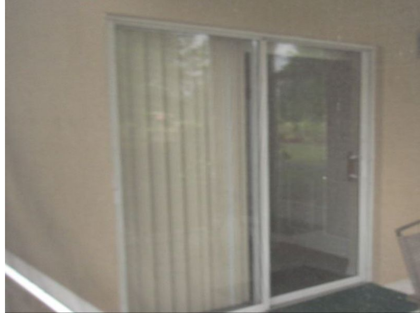
Unprotected Glazed Entry Door
