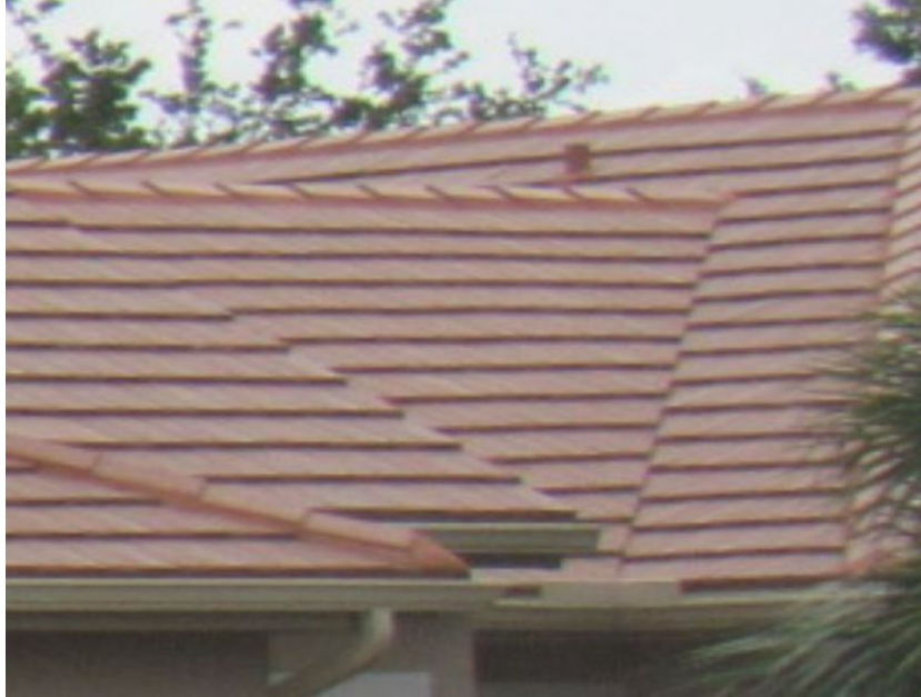
Concrete/Clay Tile Roof Covering
