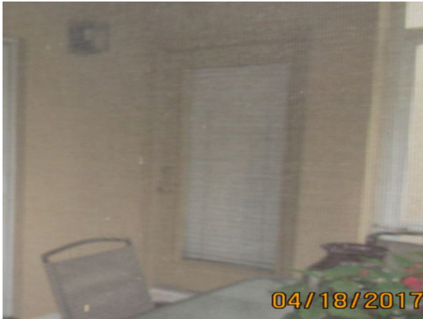
Unprotected Glazed Entry Door
