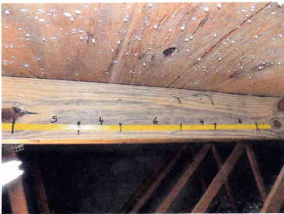
Roof Deck Nail Spacing 6"
