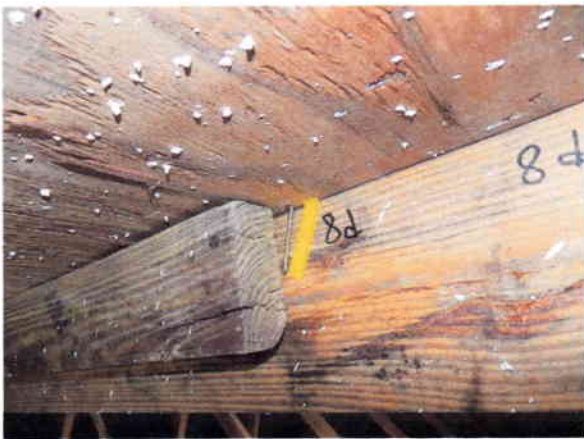
Roof Deck Attachment 8d
