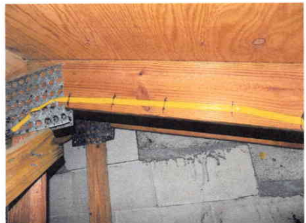
Roof Deck Nail Spacing 6"
