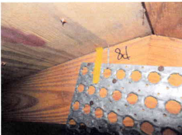
Roof Deck Attachment 8d
