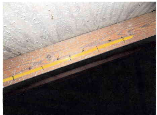
Roof Deck Nail Spacing 6"
