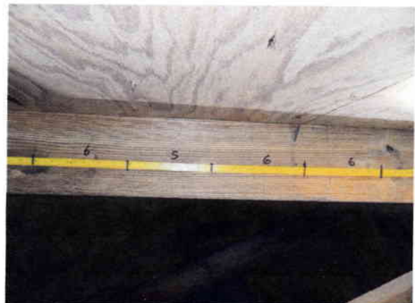
Roof Deck Nail Spacing 6"
