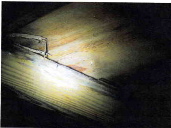
Roof Deck Attachment 8d
